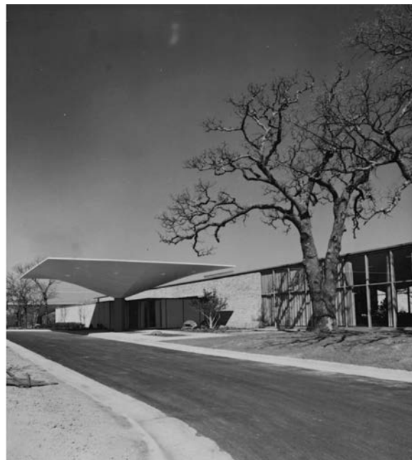
Edificio en el Parque Industrial de la Great Southwest Corporation, Arlington, Texas, con el acceso enmarcado y protegido por un paraguas, 1958. O'Neil Ford & Associates (Richard Colley, Arch Swank y Sam Zisman), consultor estructural: Félix Candela. Foto: Félix Candela Architectural Records and Papers, Dept. of Drawings & Archives, Avery Architectural and Fine Arts Library. Columbia University.
