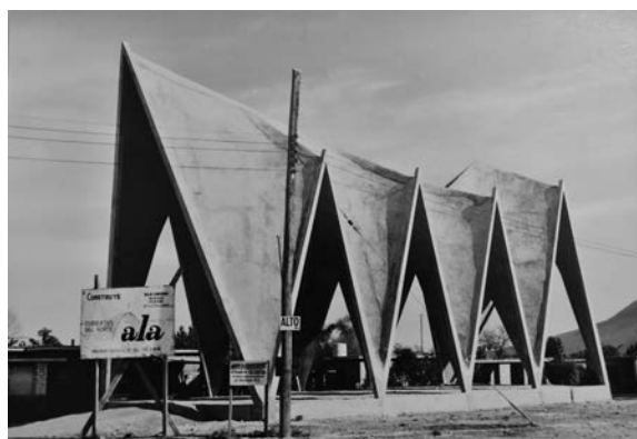
Capilla de Santa Teresita del Niño Jesús, en obra, colonia Churubusco, Monterrey, N. L., 1961. Foto: Félix Candela Architectural Records and Papers, Dept. of Drawings & Archives, Avery. Architectural and Fine Arts Library. Columbia University.
