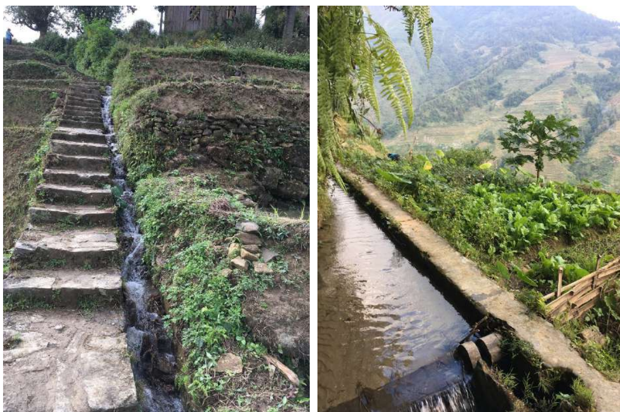
Figs. 12-13: Irrigation system of the rice terraces (Thibault, 2019)
