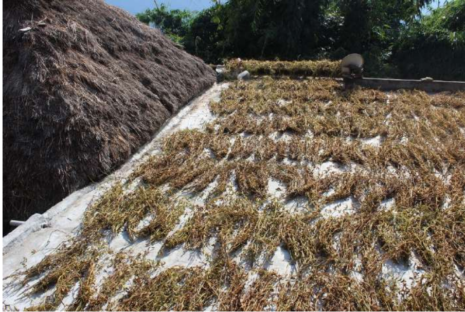
Fig. 6: Flat roof with beans drying (Martin, 2019)
