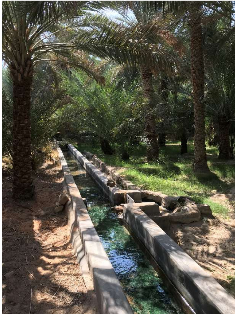
Fig. 4: Ancient technology with modern materials – concrete walls of the tributary channels ( awamid ) and plastic sluices for today's afraj (Wigboldus, 2018).
