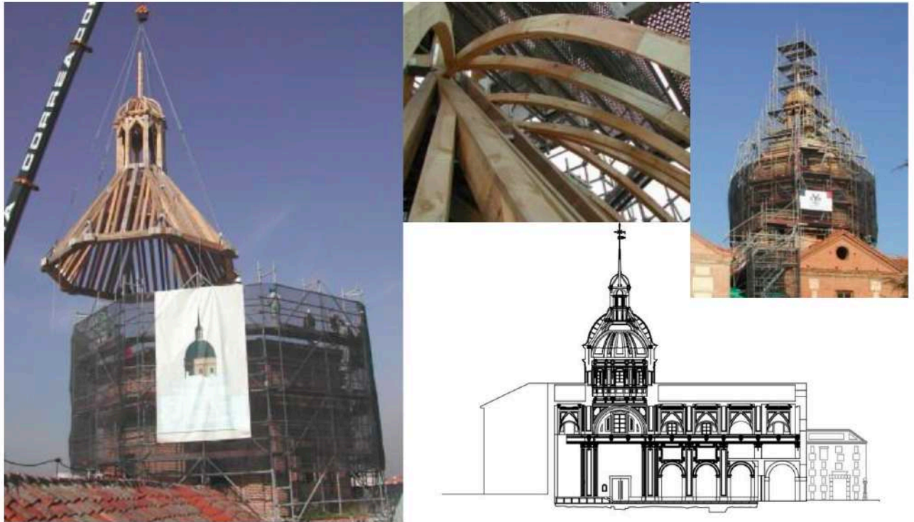
Longitudinal section and placement of the dome
