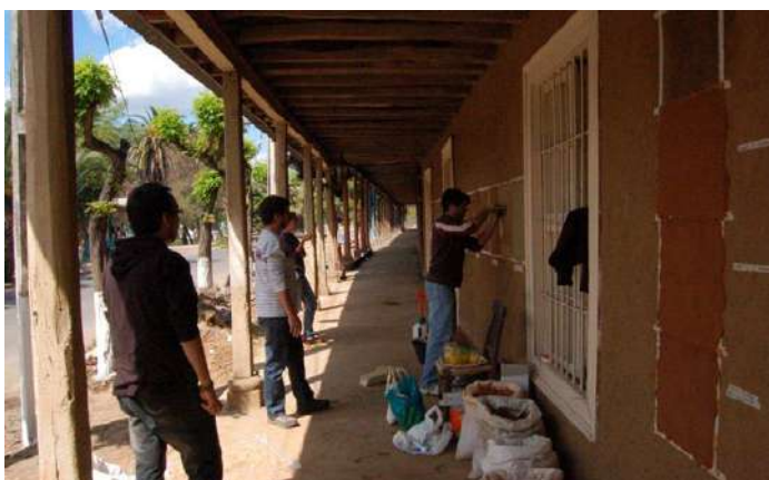
Fig. 27. Workshop in applying mud stucco, Quinta de Tilcoco, San Pedro de Alcántara, O'Higgins region, Chile (Source: SEREMI, MINVU)
